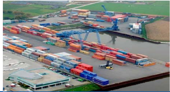
Terminal Overview Venray Barge Terminal:
