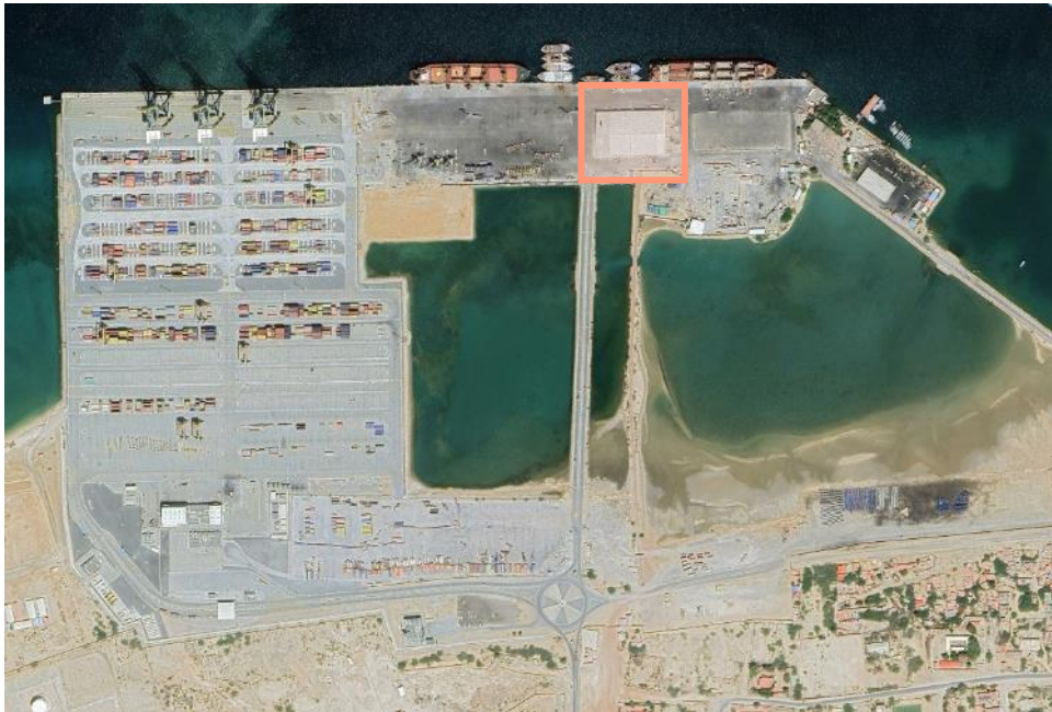
Figure 14. Berbera Port in Somalia (grain warehouse in the top-right part)
