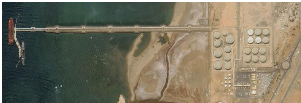
Figure 20. Horizon Terminal at the Djibouti Port
