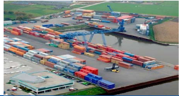
Terminal Overview Venray Barge Terminal:
