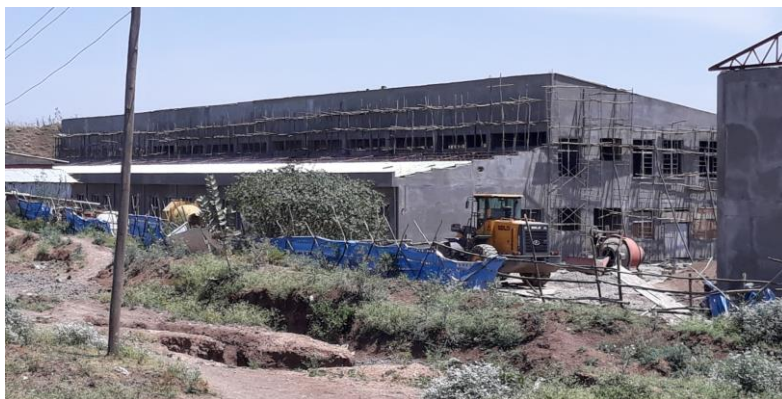
Figure 26: Construction Site of New Workshop
