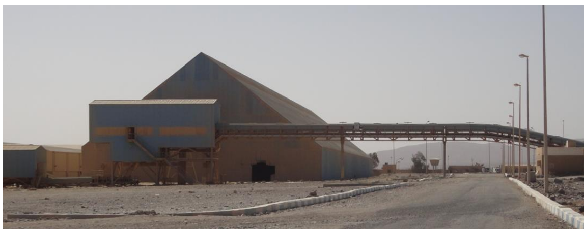
Figure 22: Example of a Fertilizer Warehouse
