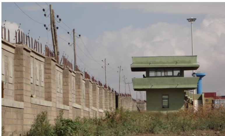
Figure 27: Watchtower and Fencing Facility of Modjo Dry Port
