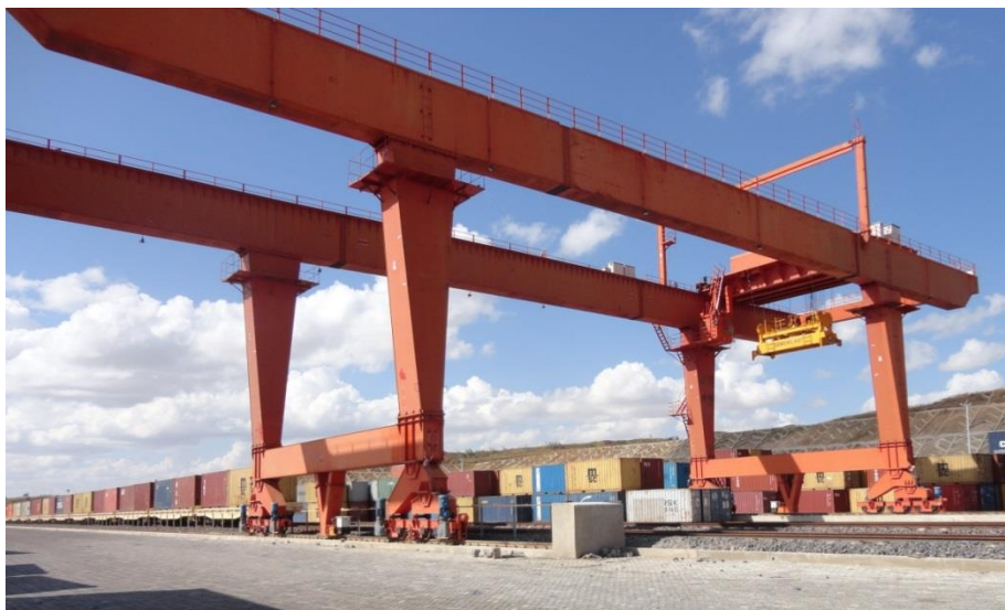
Figure 23: Current Location of the RMG Rail Yard Crane
