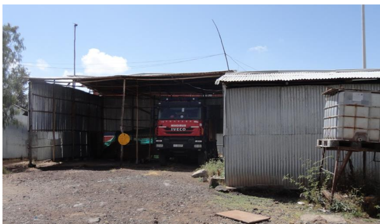
Figure 29: Current Fire Brigade Station
